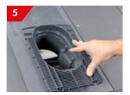
Slide the vent - spigot first - into the opening. Using the centring line on the vent, align with the joint line of the two slates directly below.
