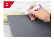
Place the adjacent slate and mark the required size to cut the slates.
