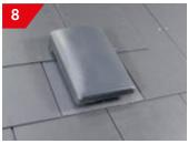
Clip the Cap of the Slate Vent securely. Continue to fix subsequent slate courses as normal. No further slate cutting is required
