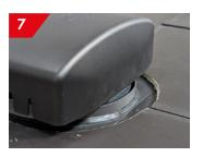
The two slates on the course above will need to be cut around the upstand of the slate vent. The slates should not touch the upstand; a 10mm gap should be maintained.
