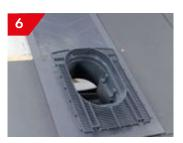
Fix vent by nailing through centre nail holes. Place the adjacent slates around the Slate Vent accordingly.
