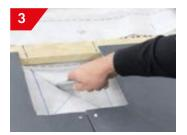
Carefully cut the underlay diagonally on the marked cross and peel back the underlay to the surrounding batten and under the slates for the sides.
