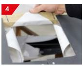
Fix the Underlay onto the batten. For rigid sarking board cut out the rectangle.
